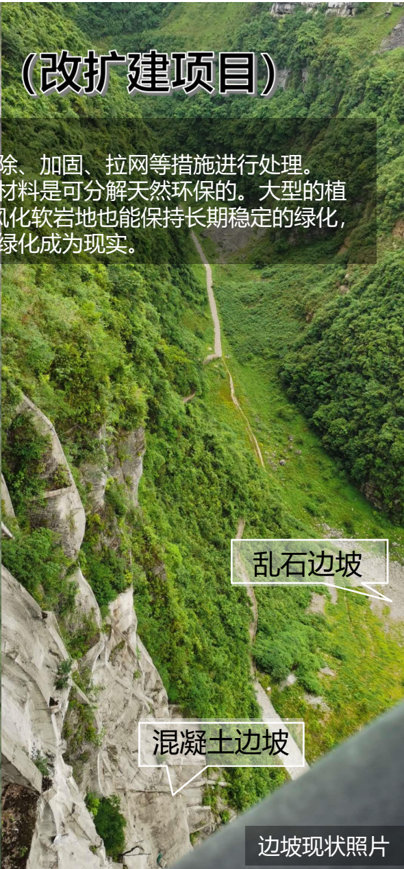
边坡现状照片
